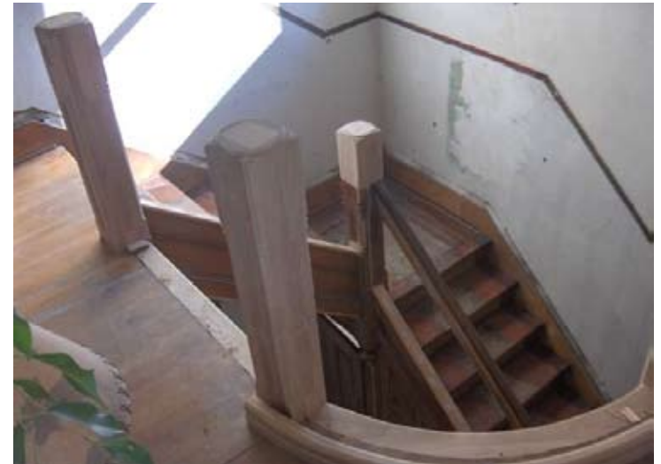
Photos left, above and below: March-June 2007. Master craftsman Matt Doneen recreated the missing oak posts and railings of the grand staircase. Doneen took meticulous measurements of the one remaining post and rail, recreated the components in his shop, then assembled the pieces on site.
