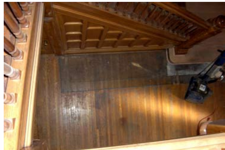
Photo above: March 2009. The tiger oak floors of both lower and upper foyers were sanded and refinished.
