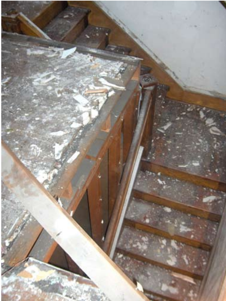
Photo above: February 2007. Some of the second floor partition wall removed revealing the treads and risers of the grand staircase.
