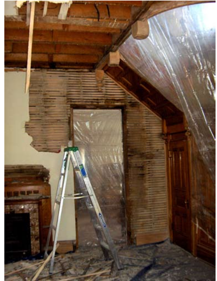
Photo above: March-June 2007. While the staircase rebuild started on the second floor, the deteriorated lath and plaster was removed directly below in the main floor foyer. New lighting, drywall and insulation was then installed.
