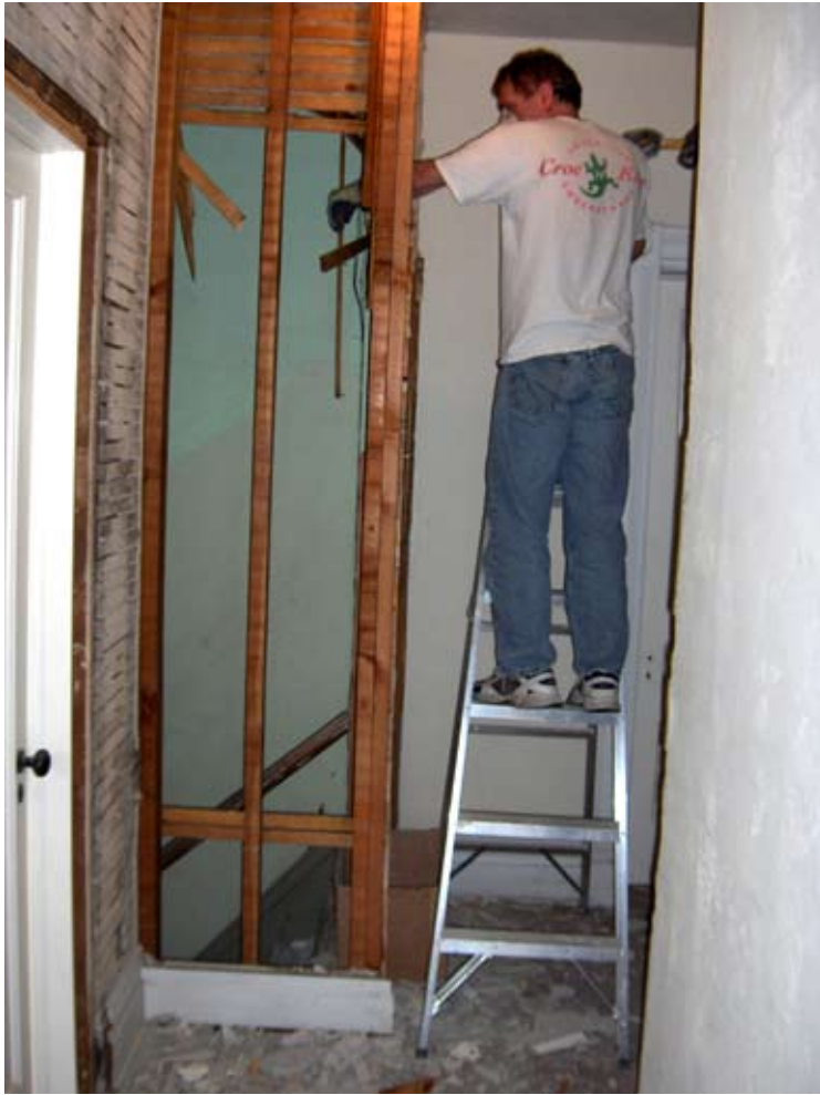
Photo above: April 2009. Steven Sanford removes lath and plaster. The maid's staircase was restored as part of the second floor hallway restoration.
