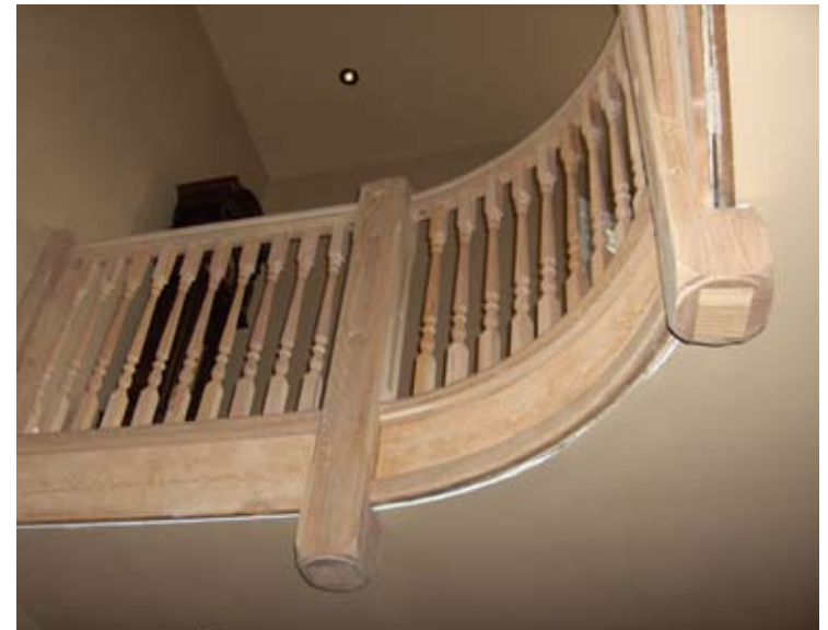
Photos left, above and below: March-June 2007. Master craftsman Matt Doneen recreated the missing oak posts and railings of the grand staircase. Doneen took meticulous measurements of the one remaining post and rail, recreated the components in his shop, then assembled the pieces on site.
